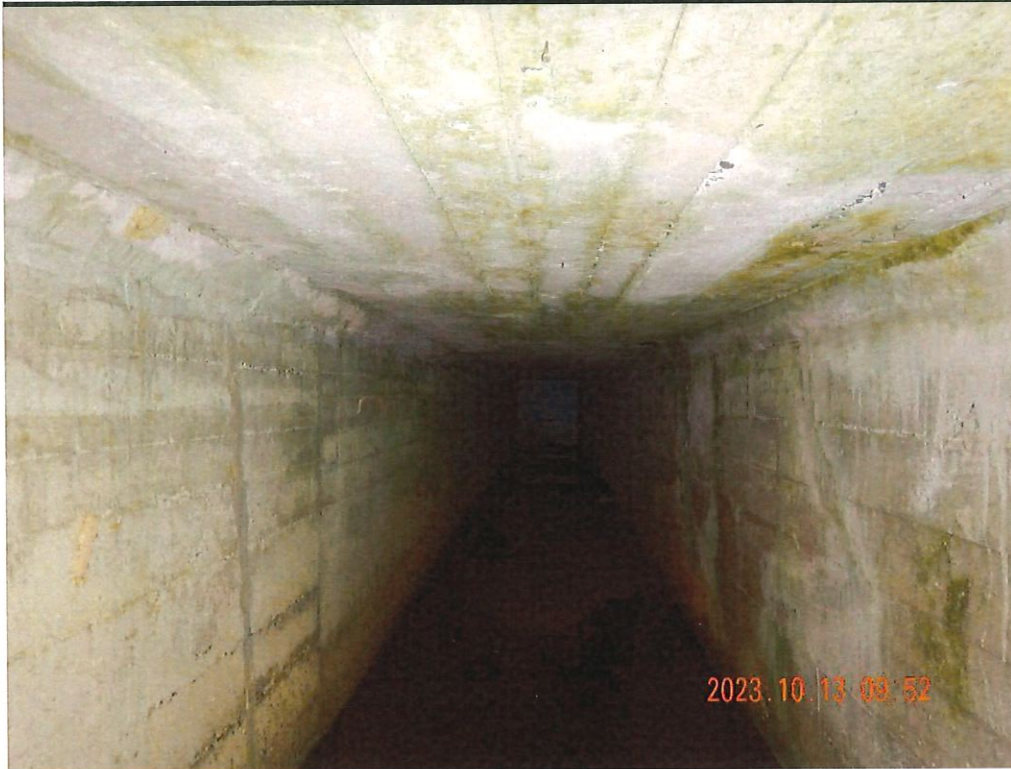
Photo 14 description: Interior Left Spillway
