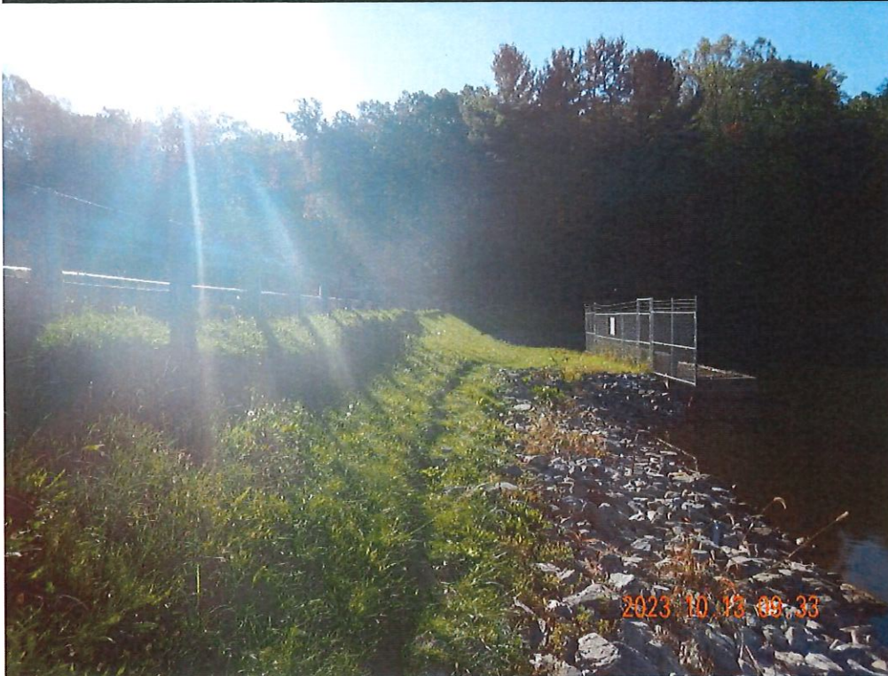
Photo 2 description: Upstream Slope Center
