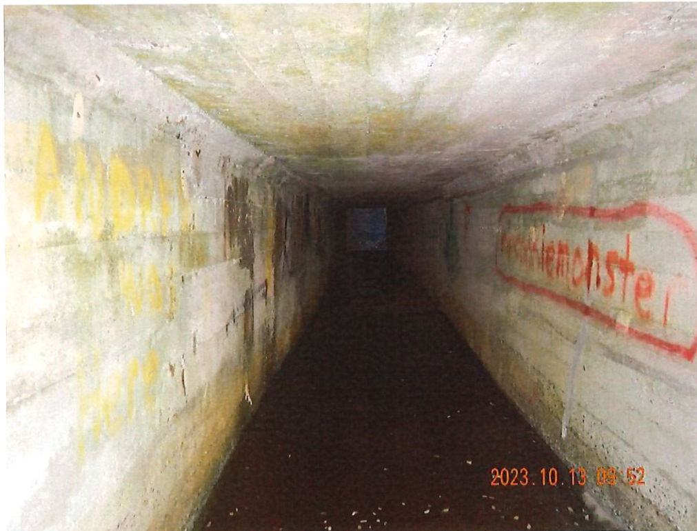
Photo 15 description: Interior Right Spillway
