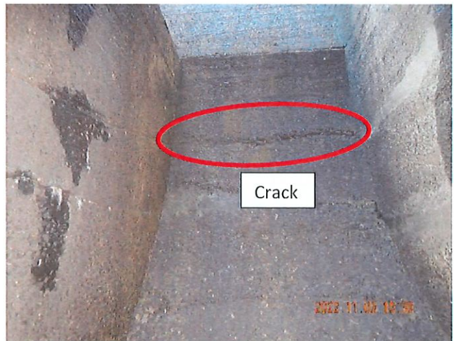
Photo 28 description: Transition Interior Right Spillway to Right Box Spillway
