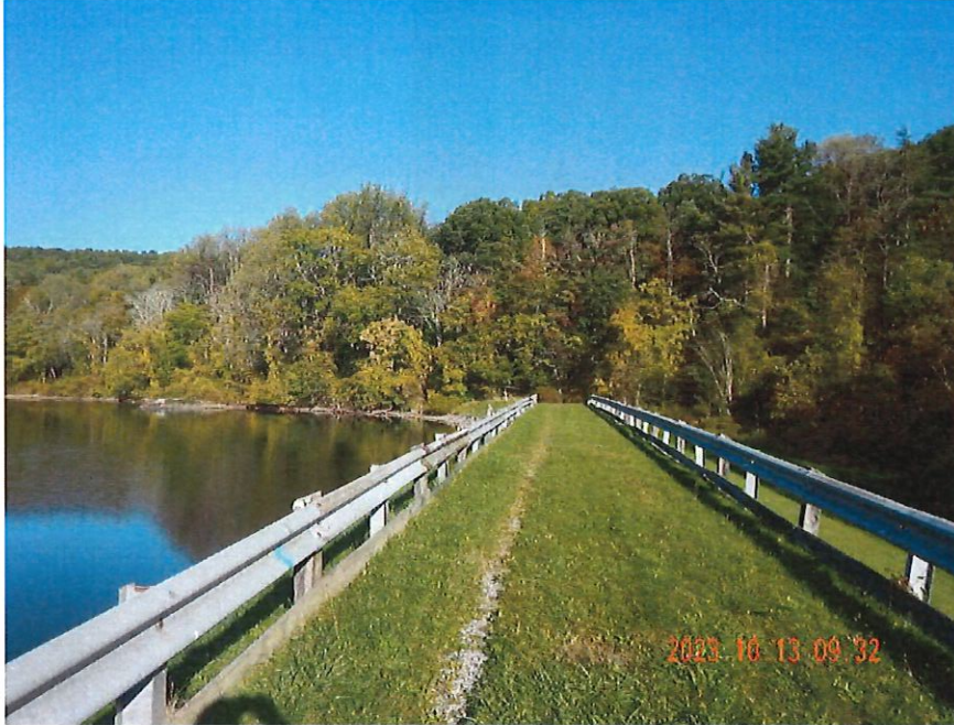
Photo 4 description: Crest Left Side
