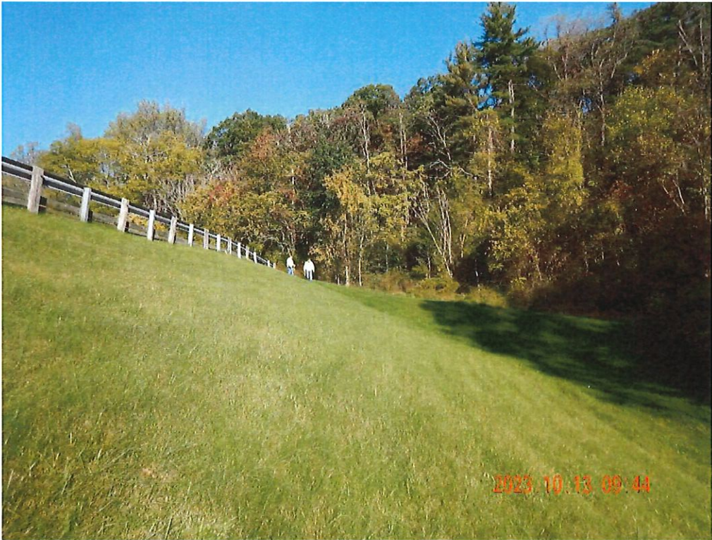
Photo 7 description: Downstream Slope Left Side
