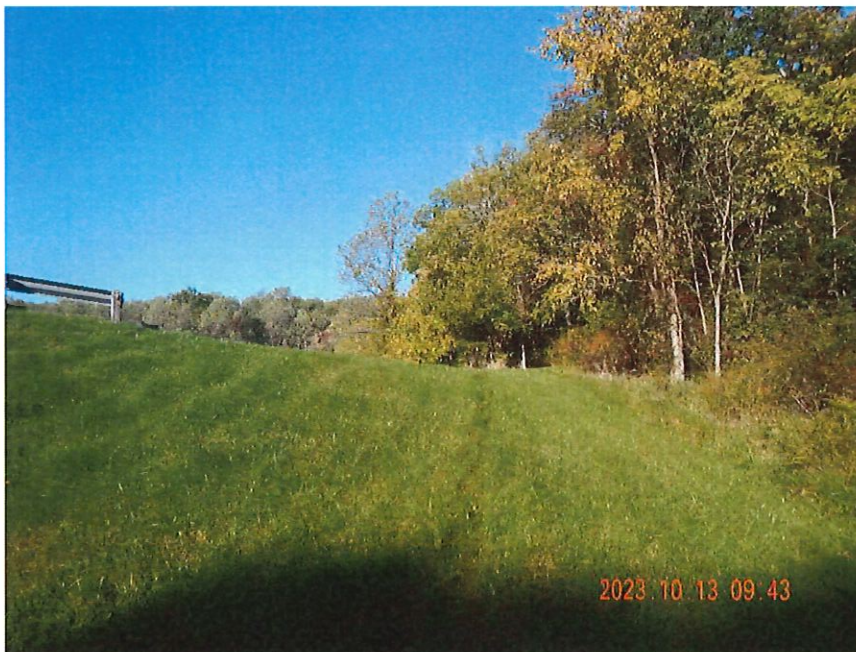
Photo 36 description: Auxiliary Spillway Exit Channel
