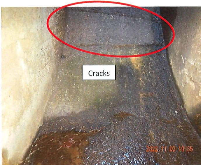
Photo 20 description: Transition Interior Left Spillway to Box Spillway
