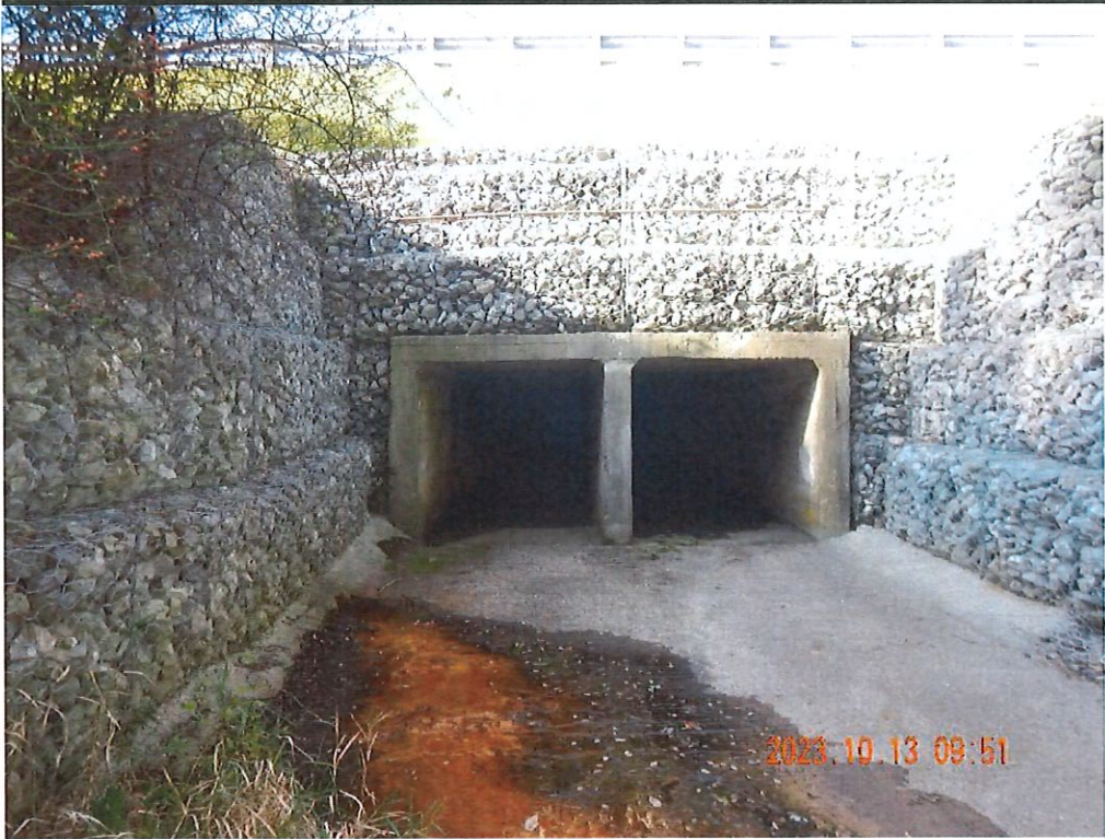
Photo 33 description: Principal Spillway Outfall/Gabion Basket Endwall
