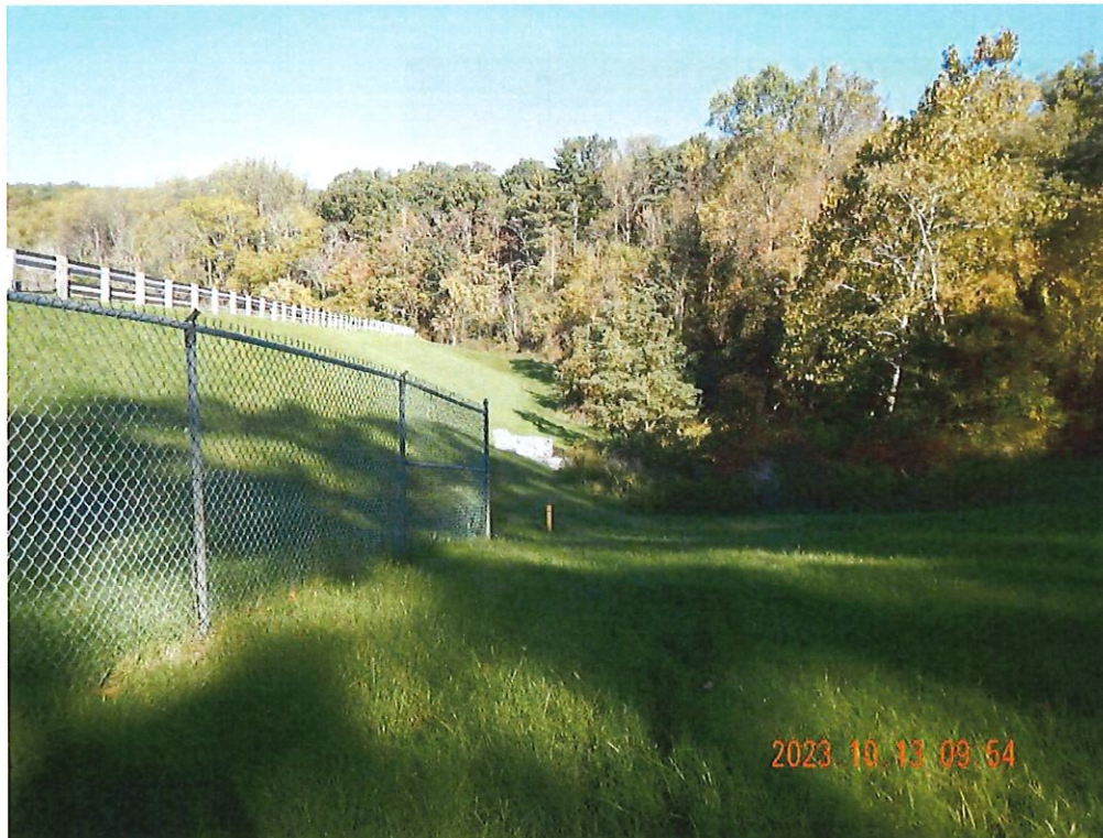
Photo 9 description: Downstream Slope Right Abutment
