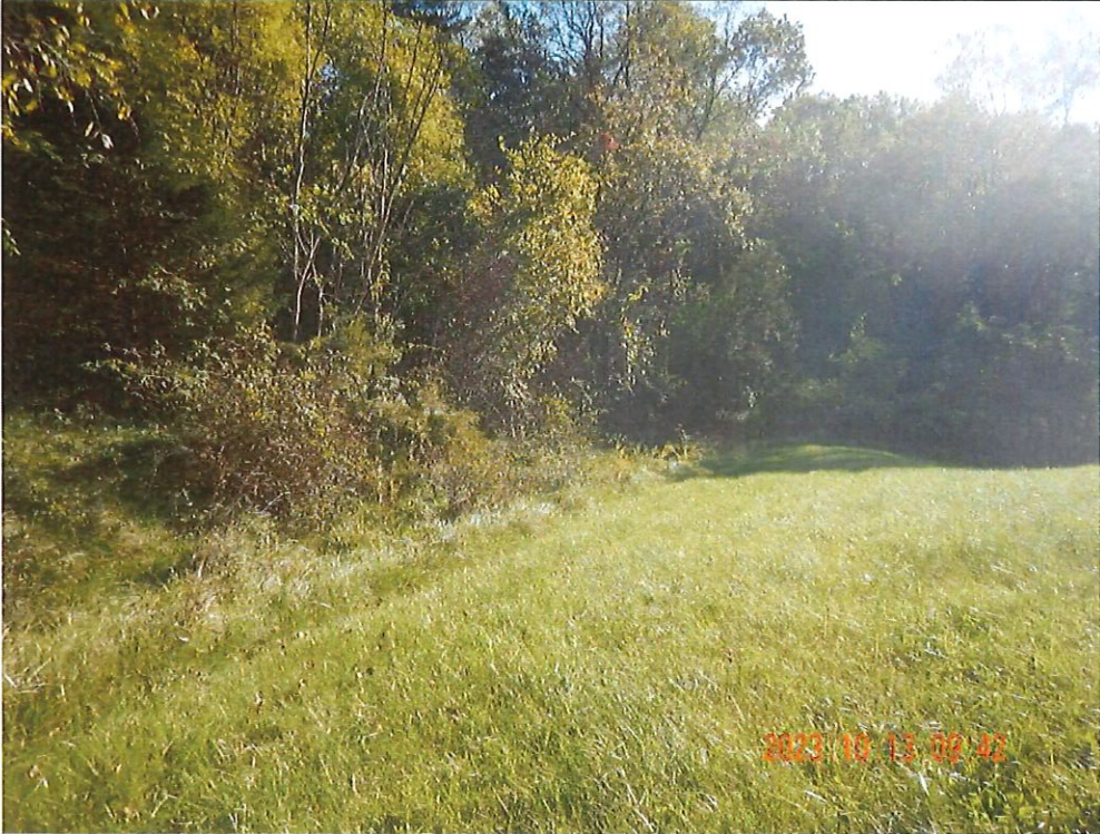
Photo 6 description: Downstream Slope Left Abutment
