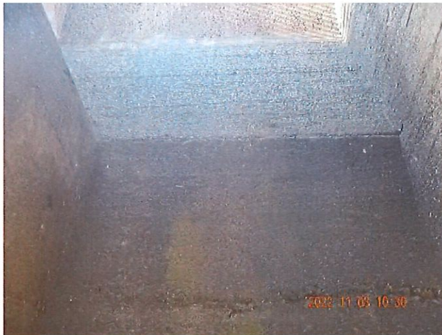
Photo 27 description: Front Side Interior Right Riser Box
