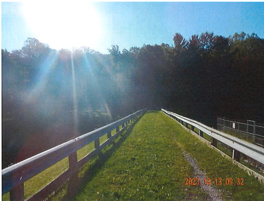
Photo 5 description: Crest Right Side
