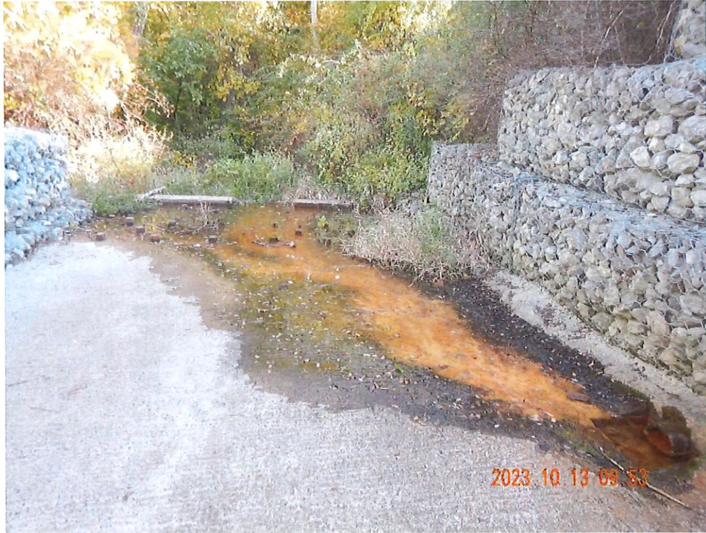
Photo 34 description: Baffle Blocks and End Sill
