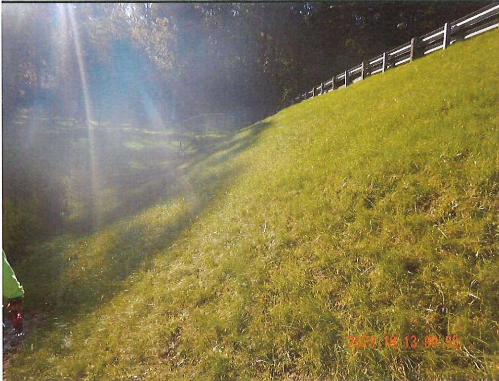
Photo 8 description: Downstream Slope Right Side
