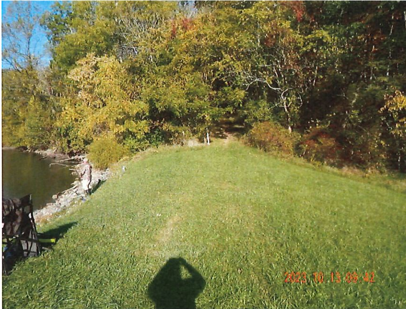
Photo 35 description: Auxiliary Spillway Control Section
