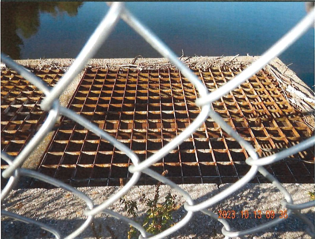
Photo 12 description: Left Gate/Weir Wall
